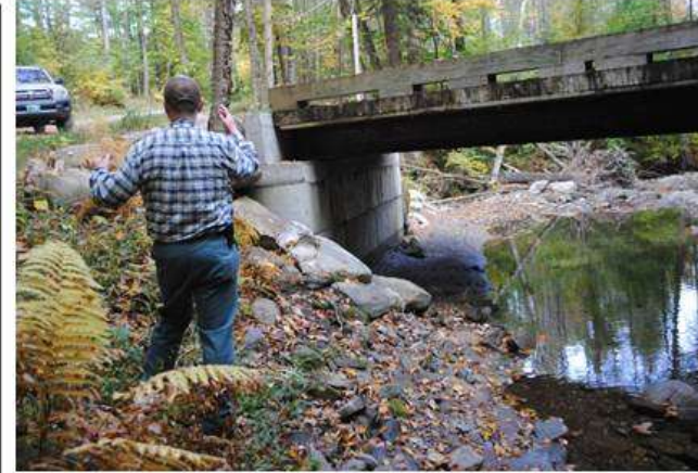
Abutment replaced after TS Irene
