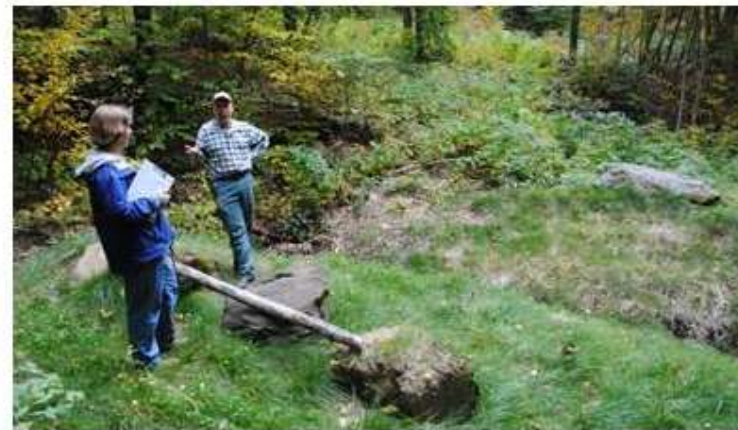
(c) Road segments have been down-sized, vegetated, and culverts removed in a portion of the access network at Curtis Hollow drainage in Coolidge State Forest East.
