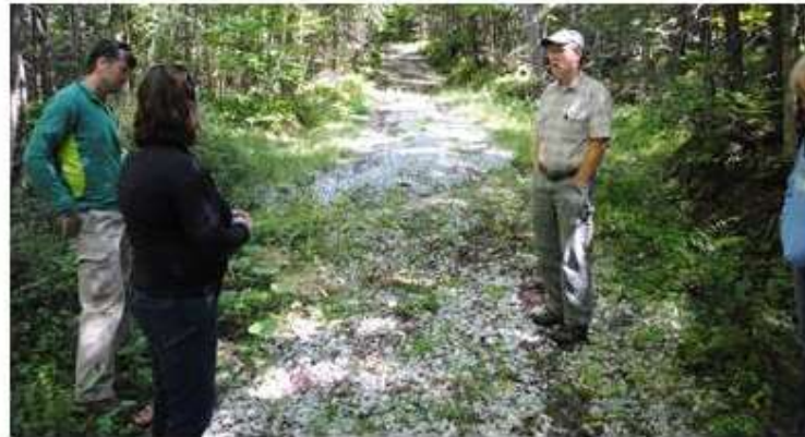
(b) broad-based dips installed on forest road in Plymbsbury WMA off Old Shrewsbury Road.
