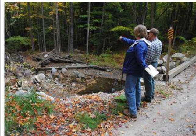
Opportunity to Disconnect Road Ditch
